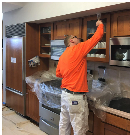
Touch-Ups A volunteer touches up the paint in the RMH kitchen. rmh.org
